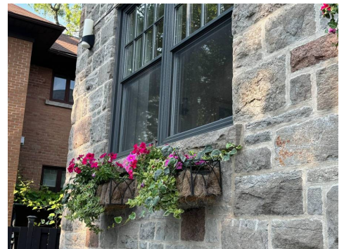
Back of building
