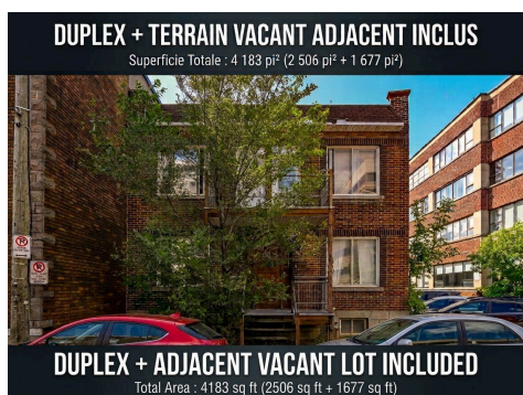
Front of building
